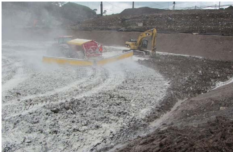
Traditional Roller Compaction
