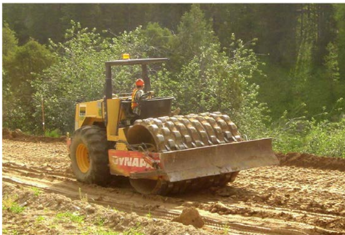
Traditional Roller Compaction
