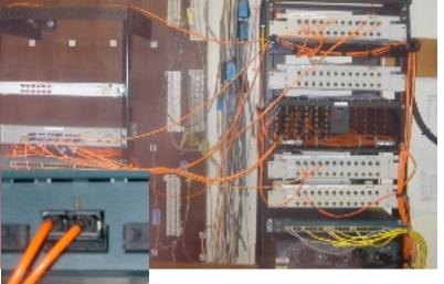
MT-RJ which has 2 fibers in one connector,
