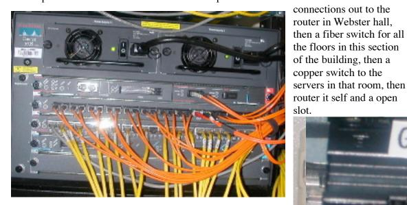
The fiber connectors are SC connector into the fiber switch, with ST connectors into the router. These 2 connectors are basically the same.(Stepanek, 2003)
