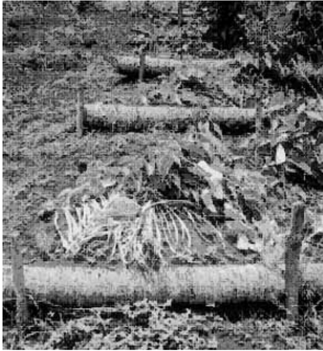
Fig. 4. Erosion control structures made of purau trunks.
